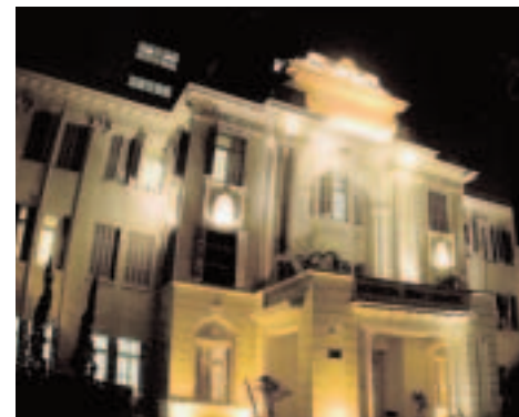
THE OLDER PART of the hospital was built in the neoclassical style of the 1920s.
