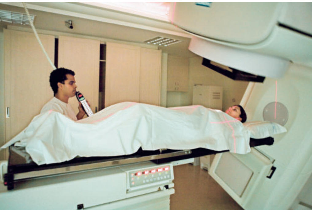
The PRIMUS Linear Accelerator not only allows Hospital Moinhos de Vento to provide fully digital radiation therapy, but was also easy to implement.
