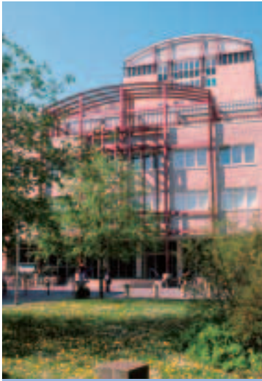
THE JOHANNES GUTENBERG UNIVERSITY HOSPITAL in Mainz, Germany, operates on IHE-based medical and information systems.
